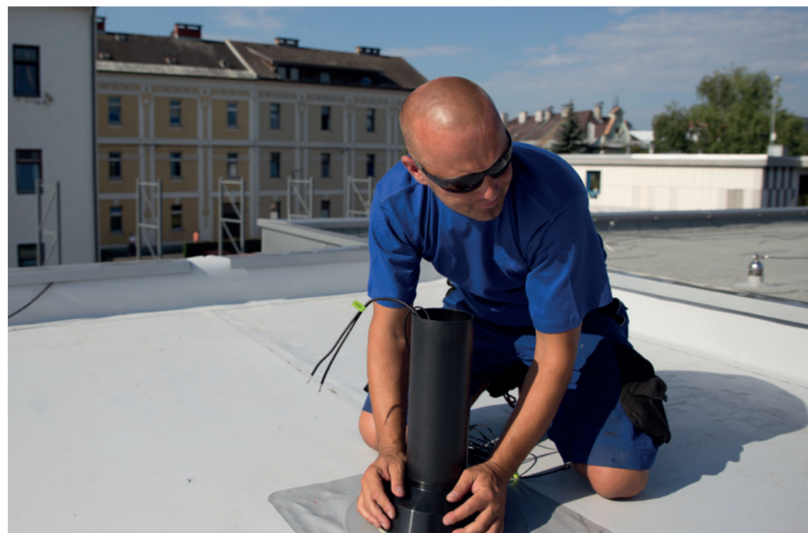
STEP 10 – FIT PIPE ON CONNECTION FLANGE
