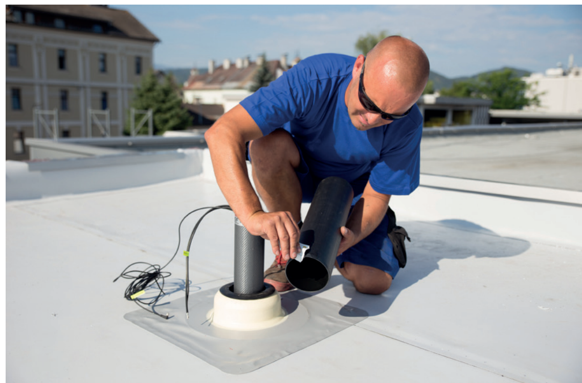
STEP 9 – FIT PIPE ON CONNECTION FLANGE
