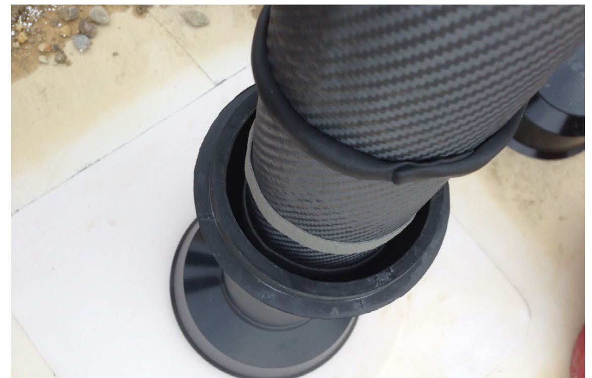
STEP 12 – INSERT ROOF PROTECTORS
