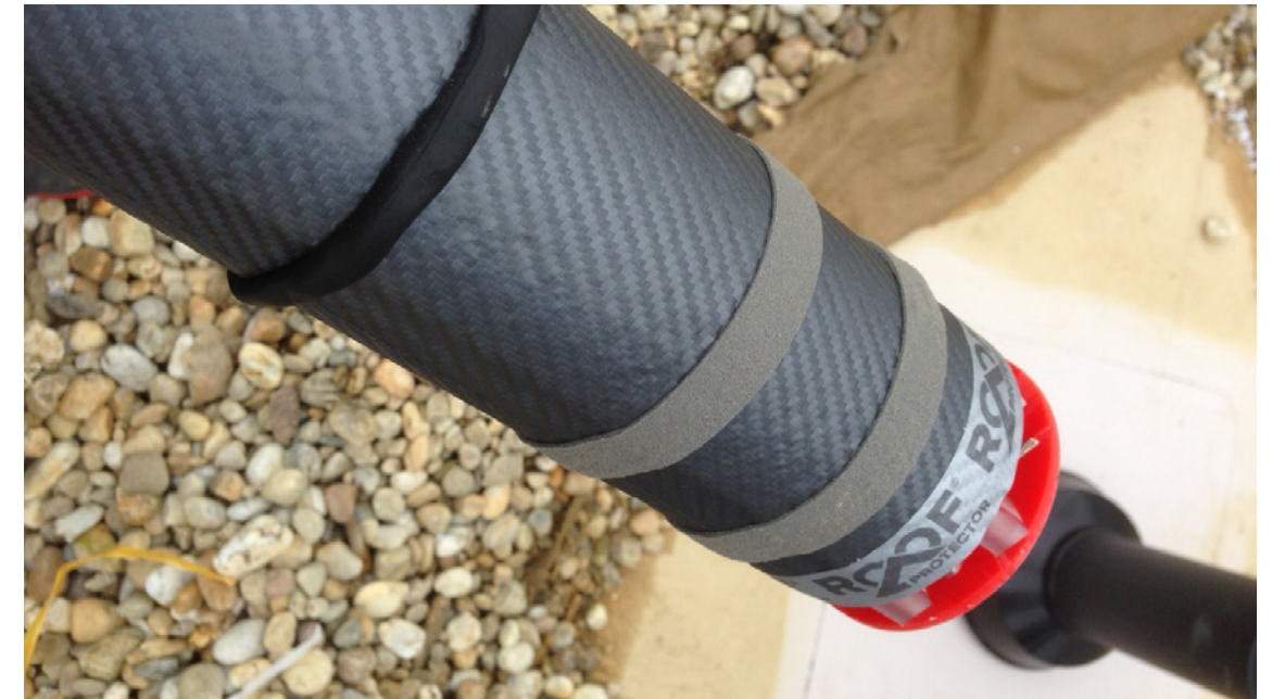
STEP 11 – SEALING USING JOINT TAPE AND ROUND BUTYL CAULKING STRIP
